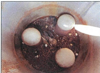
Picture No.58 : Visual inspection and remove scale on IP steam drum silencer
