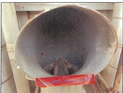
Picture No.47 : Visual inspection and remove scale on flash tank silencer
