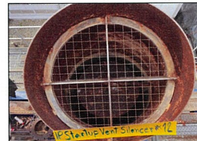
Picture No.67 : Visual inspection and remove scale on IP startup vent silencer
