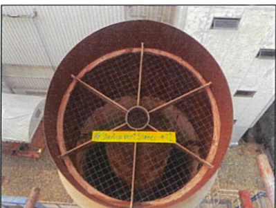
Picture No.72 : Visual inspection and remove scale on HP startup vent silencer
