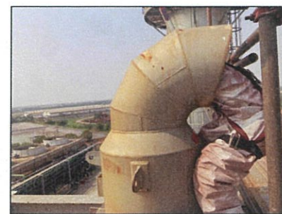
Picture No.62 : Visual inspection and remove scale on deaerator silencer
