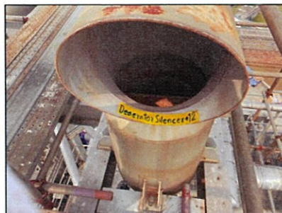
Picture No.78 : Visual inspection and remove scale on Deaerator silencer
