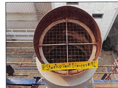
Picture No.69 : Visual inspection and remove scale on IP startup vent silencer
