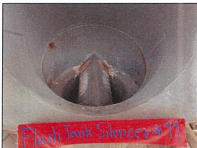
Picture No.46 : Visual inspection and remove scale on flash tank silencer
