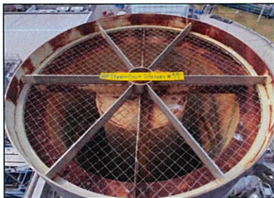
Picture No.76 : Visual inspection and remove scale on HP steam drum silencer
