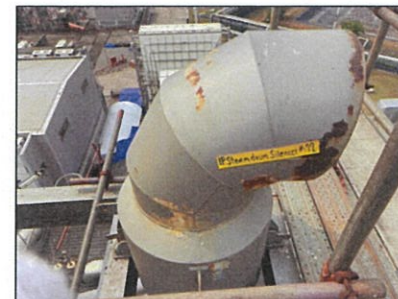
Picture No.73 : Visual inspection and remove scale on IP steam drum silencer
