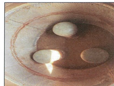
Picture No.75 : Visual inspection and remove scale on IP steam drum silencer
