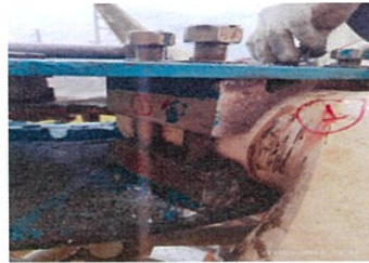
Remove Fanblade For Coating
