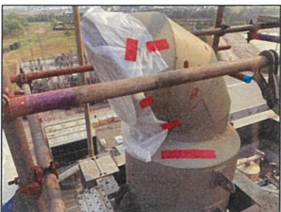
Picture No.60 : Visual inspection and remove scale on IP steam drum silencer
