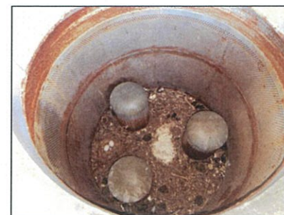
Picture No.74 : Visual inspection and remove scale on IP steam drum silencer
