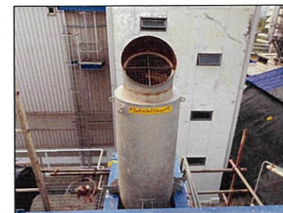
Picture No.68 : Visual inspection and remove scale on IP startup vent silencer
