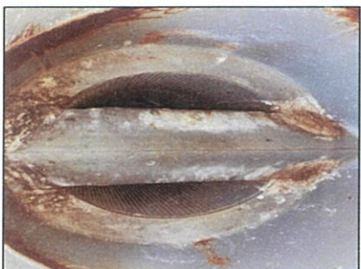
Picture No.48 : Visual inspection and remove scale on flash tank silencer
