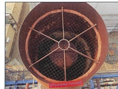
Picture No.49 : Visual inspection and remove scale on HP startup vent silencer
