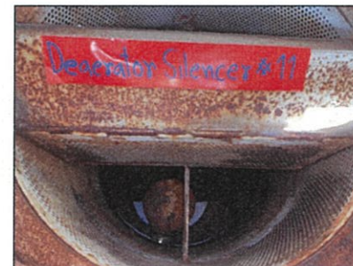
Picture No.61 : Visual inspection and remove scale on deaerator silencer
